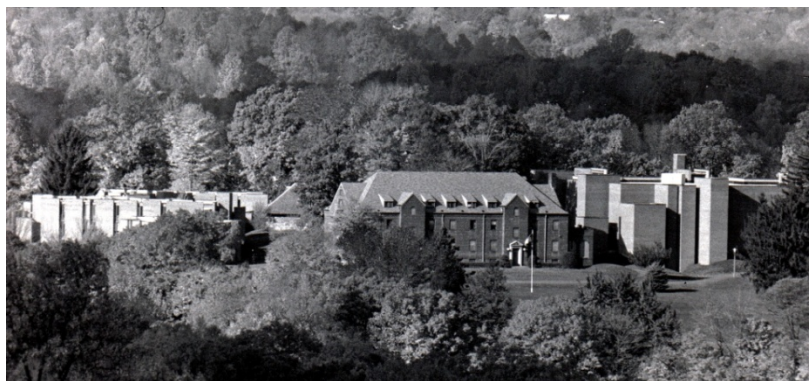
42 SMA Monastery Complex
